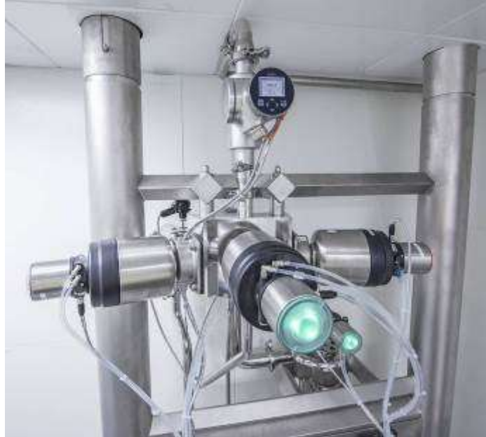
Fig.10 FLOWave sensor mounted on the pneumatic conveyor (Bürkert, 2020)
