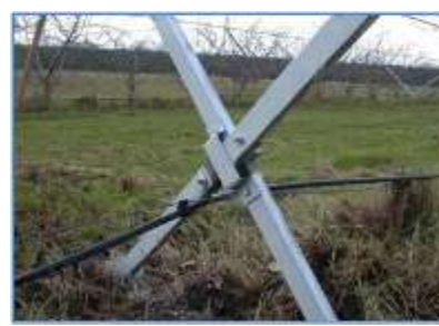
Figure 9. Joint between trellis beams
