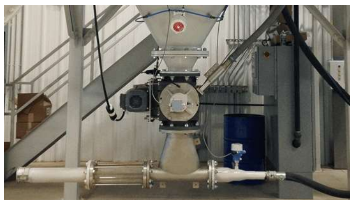
Fig.9 High Pressure Rotary Valve
