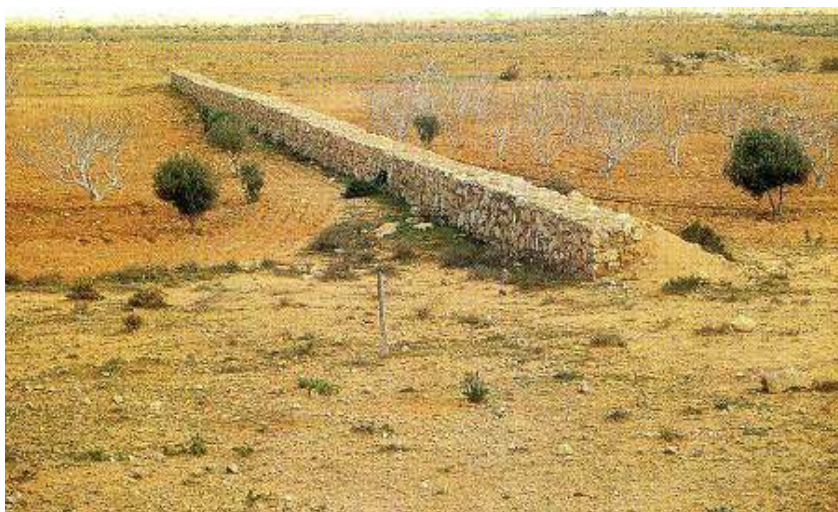
Fig. 6. Wadi-bed Cultivation Water Harvesting System for Erosion Control
